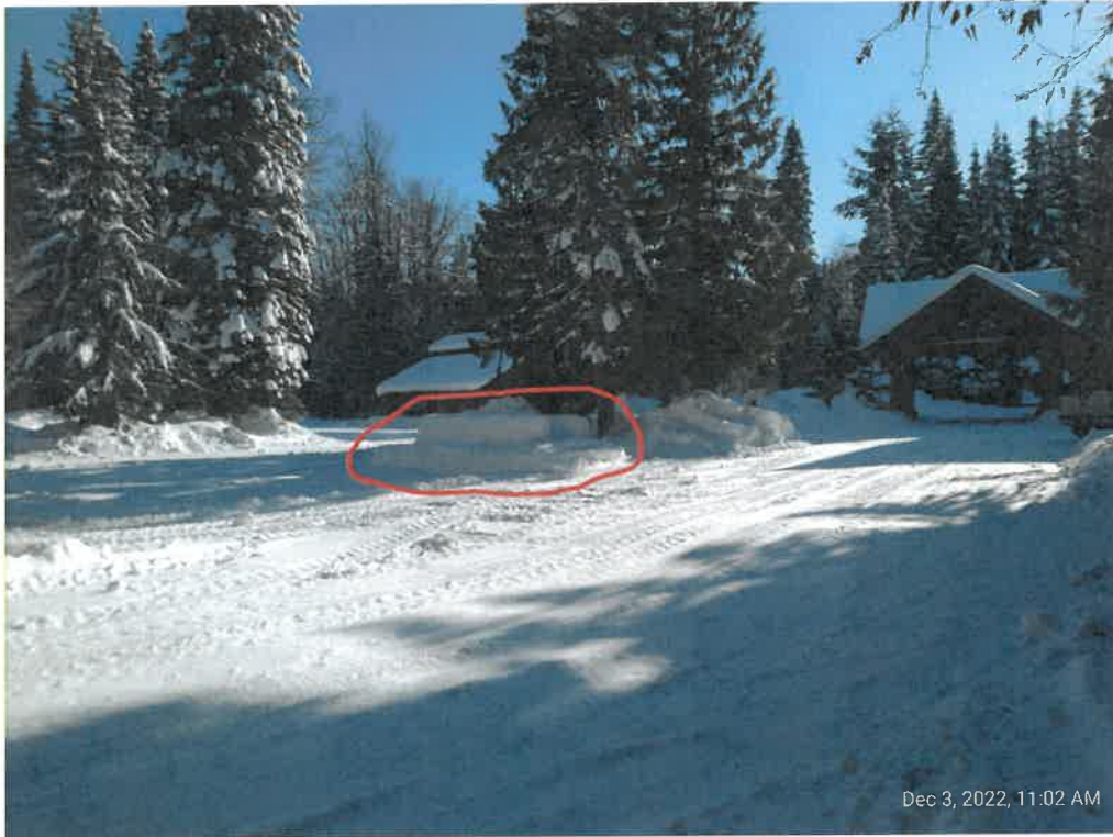
Figure 2. Propane tanks in the middle of the parking lot.
